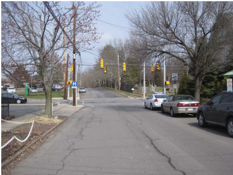
Intersection 1 - Courtright Avenue Looking Westbound at 100'
