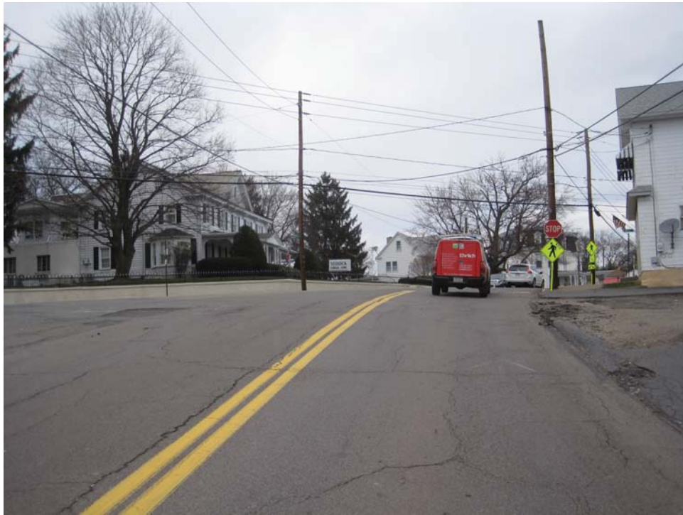
Intersection 9 – SR 2022 Looking Northwestbound at 100'
