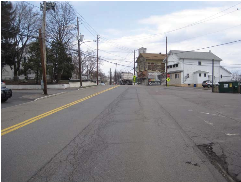
Intersection 9 – SR 2024 Looking Northbound at 100'
