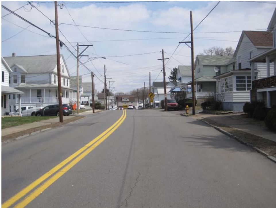
Intersection 7 – SR 2024 Looking Northbound at 100'
